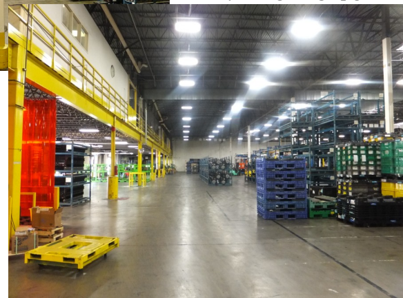
After lighting upgrade
