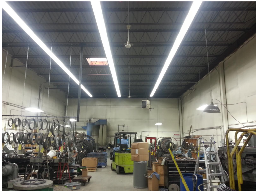
Marshall Spring Manufacturing – after lighting retrofit
